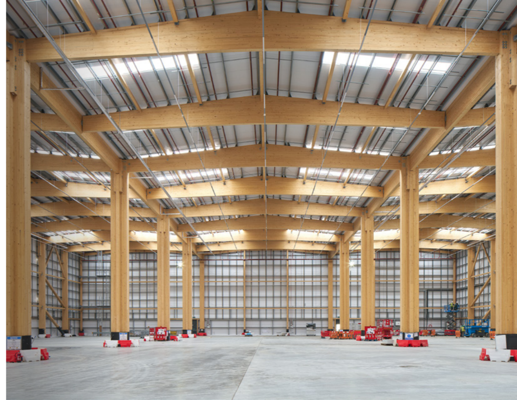
Left Ireland's first Net Zero Carbon logistics building at Quantum Logistics Park
